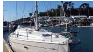
Connection of lighting points on a sailing boat (New Zealand). Series TH387.
